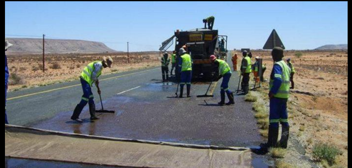
South Africa: Rehabilitation of Mpumalanga road
